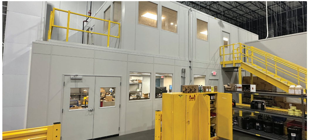
Two-Story Office with Mezzanine Structure
