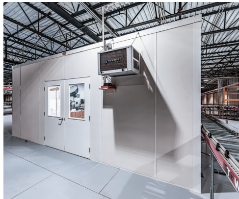
Process Enclosure with Conveyor System Integration
