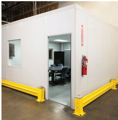
Climate-Controlled Break Room
